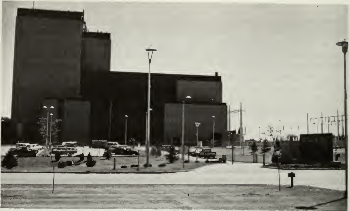
The Fort St. Vrain Nuclear Power Plant is the first and only nuclear electrical generation plant in Colorado. A. E. Turner Photo, Courtesy USGS.
